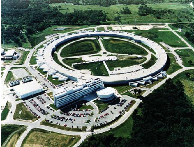
Figure 2. Aerial view of the Advanced Photon Source at the Argonne National Laboratory, Illinois, the premier third-generation synchrotron radiation facility in the United States. Photo from http://aps.anl.gov/aps/frame_home.html
