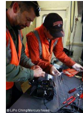
Fig. 1. Crew splicing fiber-optic cables.
