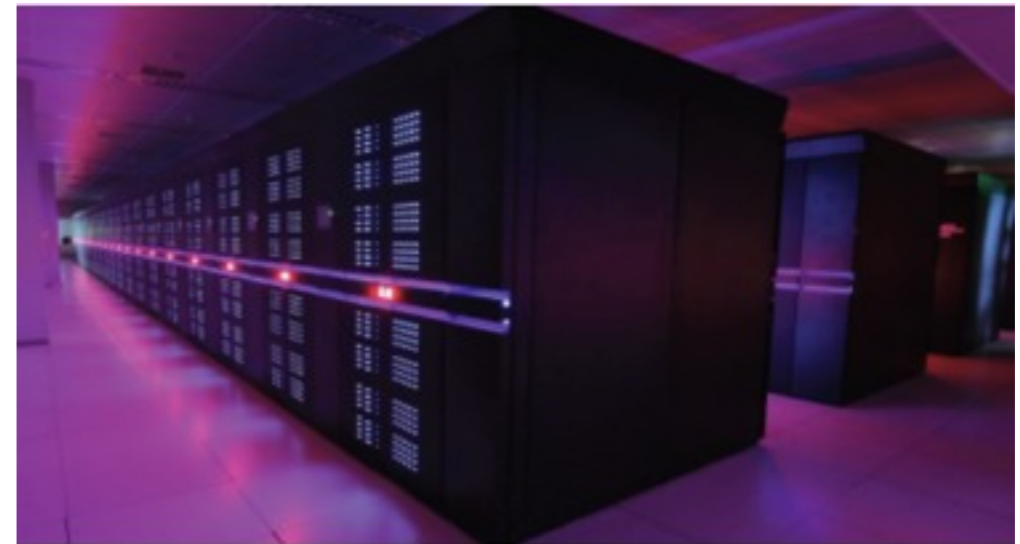
Tianhe-2 (China) (> 3 million cores)
